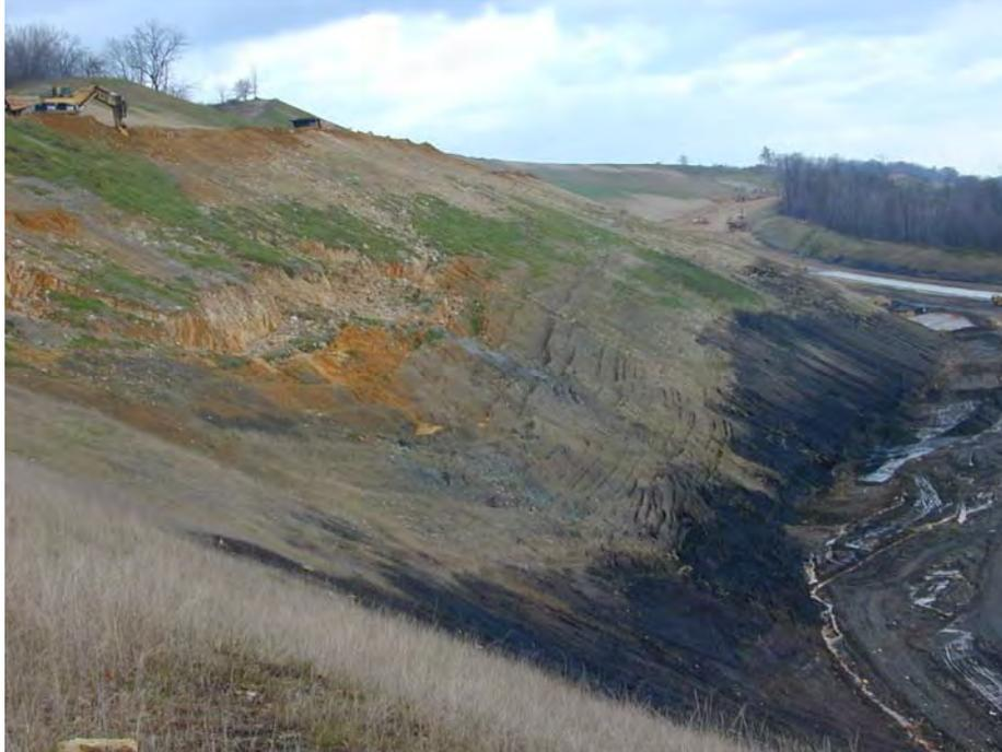
**Figure 6.** Slope failures at the US Route 22-522 Industrial Drive Interchange. Failures occurred after heavy rains associated with Hurricane Ivan had passed through the area. Construction for the Lewistown Bypass appears in the background of the photograph, and construction for the off-ramp to Industrial Drive appears in the foreground. The view is to the northeast from the southwest edge of the off-ramp roadcut. From McElroy, 2006.
