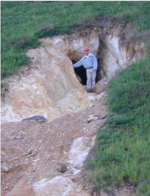
**Figure 9.** Uncovered entrance to a Ridgeley sand mine encountered during excavation.
