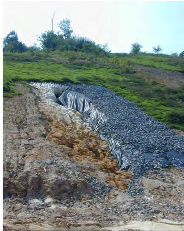
**Figure 10.** Mine opening with blown out cover.
