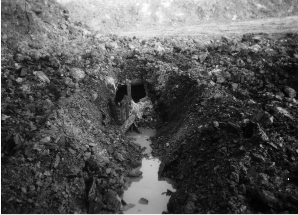
**Figure 8.** Acid drainage flows out of an old iron mine in the Marcellus Formation at the excavation site. Photograph by Fred Waldner, Site-Blauvet Engineers, Inc., 2003.
