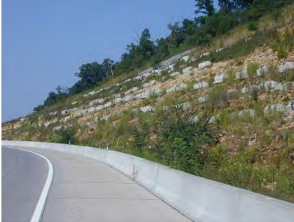
**Figure 20.** Rock anchors at mileage 4.70.
