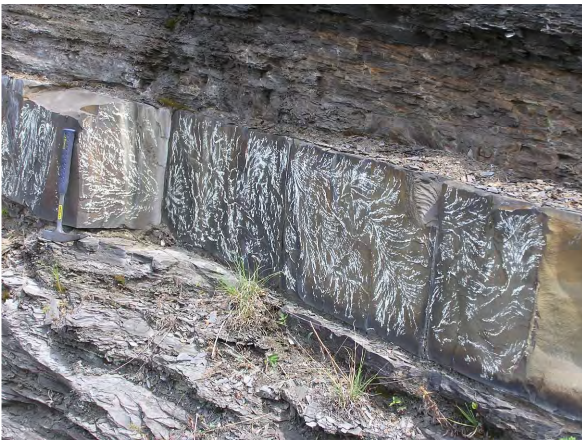
Figure 6-2. Joints in interbedded siltstone of the Brallier Formation in a road cut along Penn Street off Route 22 in Huntingdon, PA. Late-stage J 2 joint abutting a strike joint (joint propagating toward hammer).
