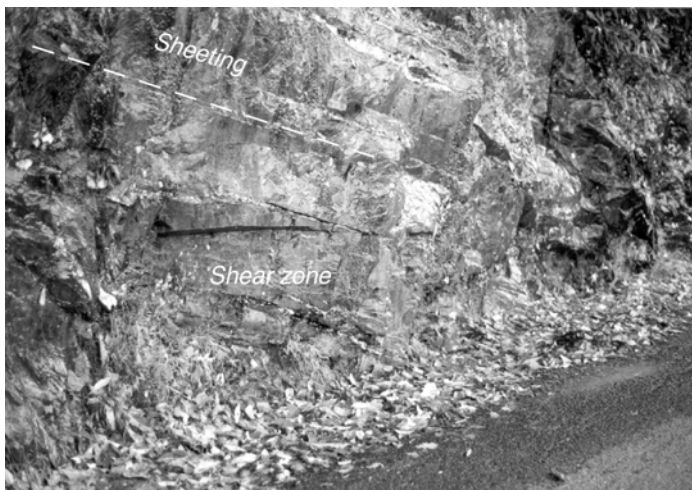
Figure 83. Sheeting joints along which the landslide along the Old Mine Road near Delaware Water Gap probably occurred. The shear zone is often wet and water seeps into the road bed below, more than is emitted from the weep pipe shown in Figure 81.
