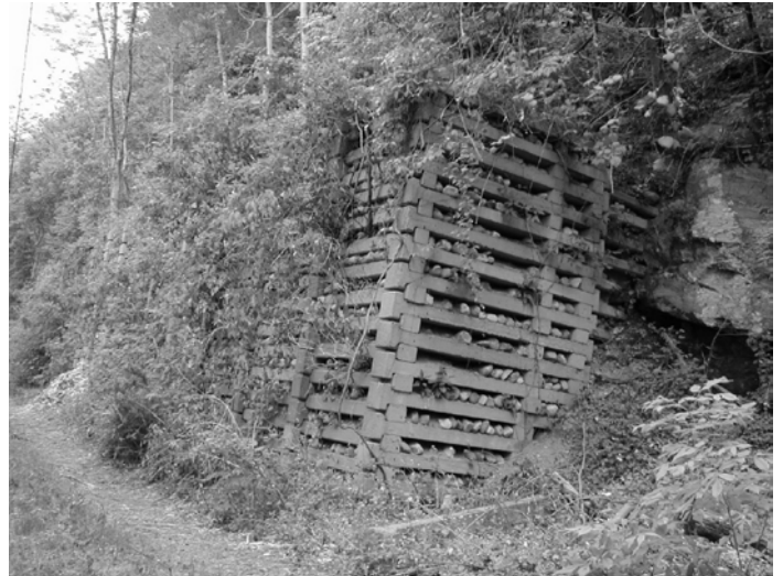
Figure 82. Concrete gabion along abandoned railroad grade below the Old Mine Road in Worthington State Park.
