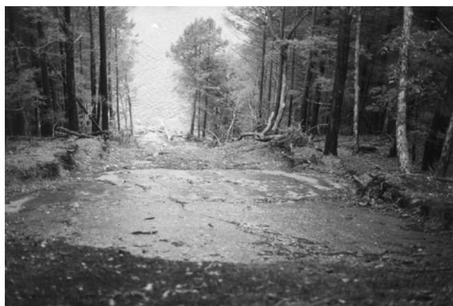
Figure 76. Initial failure area at the top of the Sambo Island landslide. This area is 37 feet wide and extends down 90 feet to a pile of debris. The bedding dips 32^\circ , paralleling the slope. The slide area extends 600 feet down to the Delaware River.
