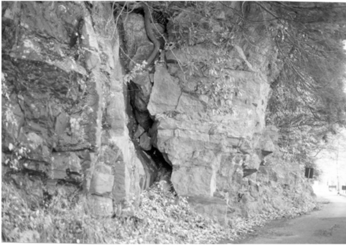
Figure 85. Irregular cross joints, trending slightly west of north and at an angle to the trend of the Old Mine Road (see Figure 84). Boulders in the fractures are wedging the block apart, creating the potential for toppling.
