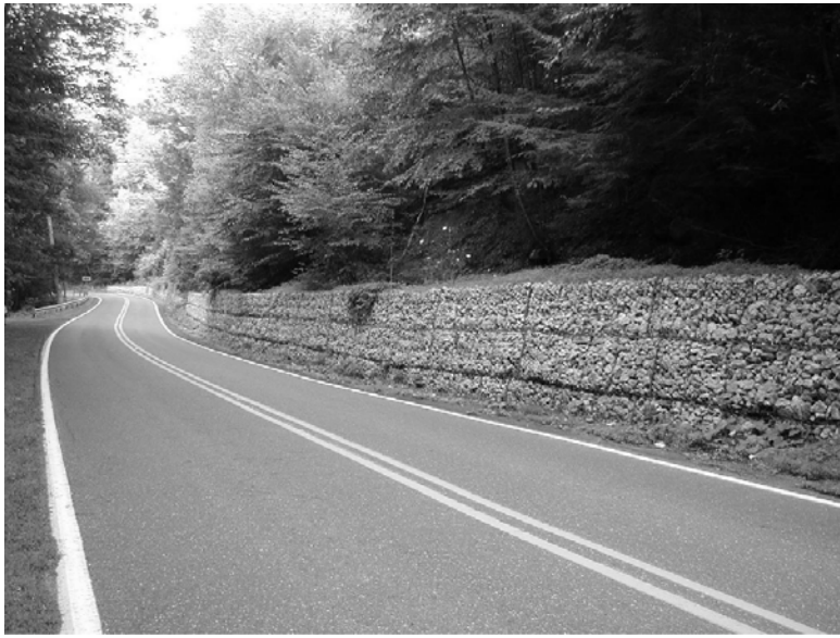
Figure 87. Gabion, about 450 feet long, along the glacial debris flow along Brodhead Road.
