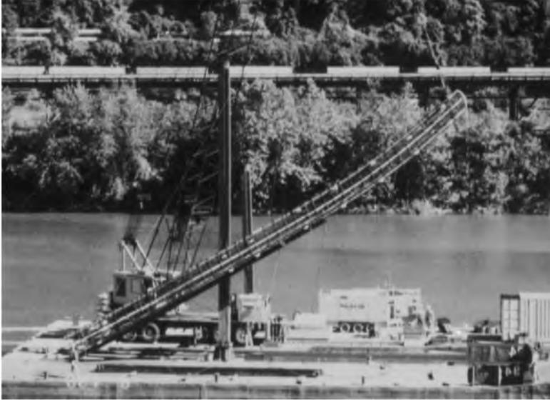
**Figure 49.** Photo of instrumented rebar cage for test shaft.
