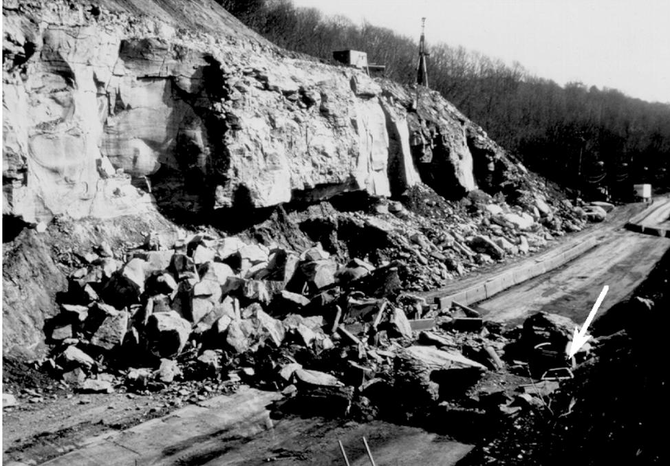
**Figure 42.** Large destructive rockfall in the undercut Morgantown Sandstone along Saw Mill Run Boulevard between the Fort Pitt and Liberty tunnels in 1983. The rockfall occurred when vibrations set up by blasting loosened a large section of the exposure. The rockfall resulted in two deaths and one serious injury. Notice the rear portion of the car protruding from beneath a large boulder-size piece of rock on the right (at arrow). Photo by Helen Delano.
