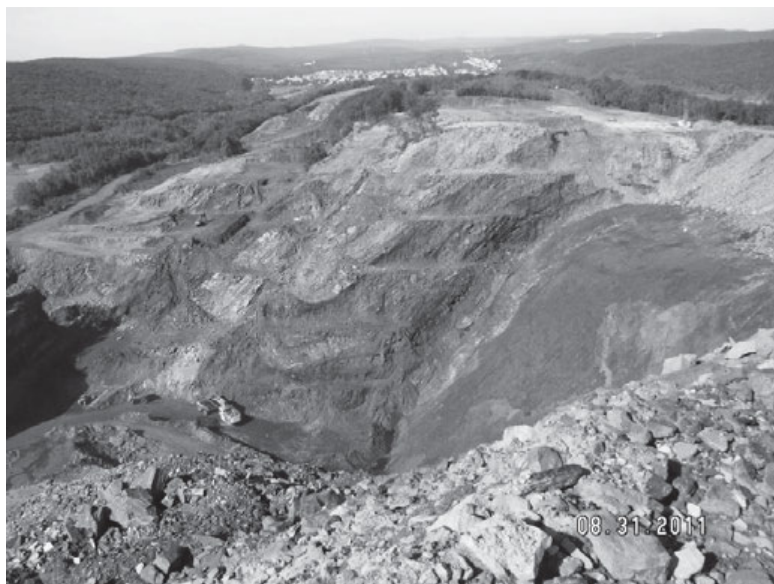
Figure 2-4. Centralia fault on the north limb of the Centralia syncline looking west. On the right is the Centralia anticline exposed by mining
