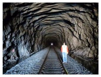
Figure 21. Unlined west part of the Erie Railroad tunnel at Otisville. The Shawangunk conglomerate here forms a ragged, but solid, arch that does not require lining.
