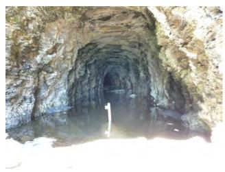
Figure 8. Close-up of the southeast portal of the O&W tunnel's east portal showing gently west-dipping bedding, water in tunnel (a constant problem during railroad operations), and lack of lining at portal.
