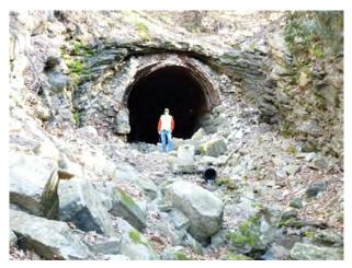
Figure 6. Northwest portal of the abandoned O&W tunnel, about 0.8 mi (1.3 km) east-southeast of Wurtsboro (GPS 41°34'00.0"N/74°28'05.7"W). Bedding in the Shawangunk conglomerate here strikes N33E and dips 26NW. Note the brick lining (with stone facing at entrance) and water flowing from pipe in foreground.
