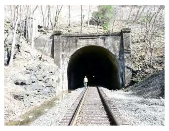
Figure 20. West portal of Erie Railroad tunnel at Otisville (GPS 41°28'41.6"N/74°33'19.9"W). Note outcrop of Shawangunk conglomerate to left of portal. The inscription reads "19—Otisville—08," the year of completion of the tunnel.
