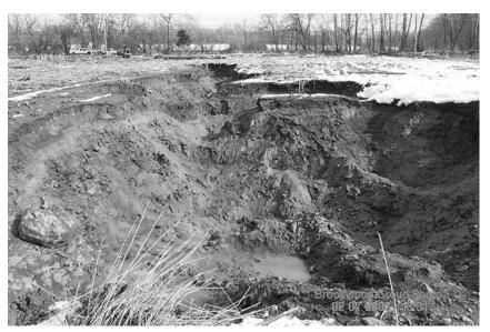
Figure 9. Drained segment of the "new" Bushkill channel. It was subsequently filled with soil and shot rock as part of the rapid response plan.
