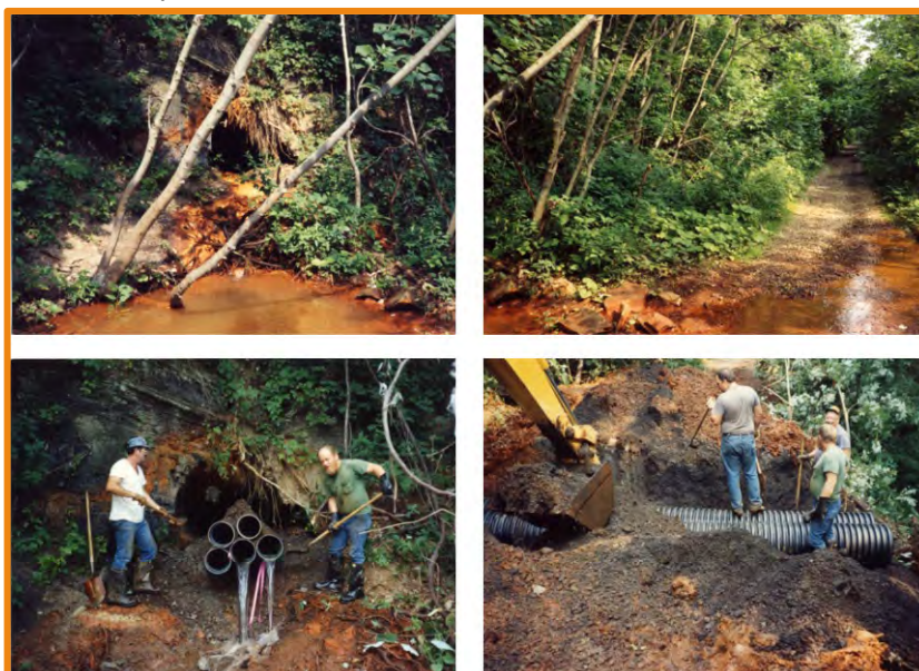
Figure 20. Photos from the pipe installation and water drainage project undertaken by BAMR in 1991 along the Great Allegheny Passage rail trail. Upper left: original Hurd mine opening. Top right: mine water flowing over and washing out the rail trail. Lower left: process of covering over outlet pipes in main entry. Lower right: installation of drainpipes under the rail trail.
