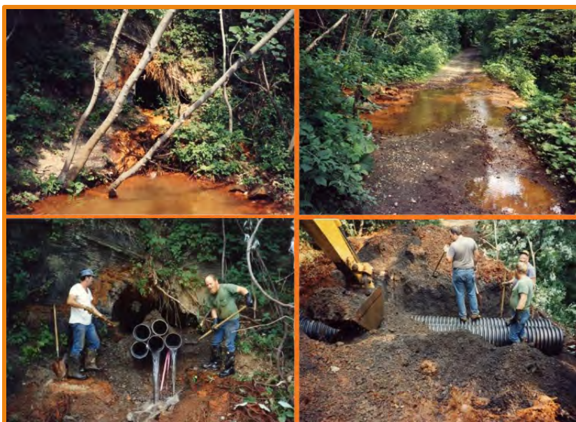
Figure 3. Photos from the pipe installation and water drainage project undertaken by BAMR in 1991 along the Great Allegheny Passage rail trail. Upper left: original Hurd mine opening. Top right: mine water flowing over and washing out the rail trail. Lower left: process of covering over outlet pipes in main entry. Lower right: installation of drainpipes under the rail trail.
